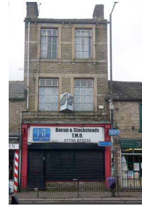
Figure 31: 27 St James Street before
