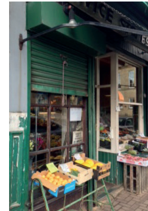
Figure 39: 7 St James Street before
