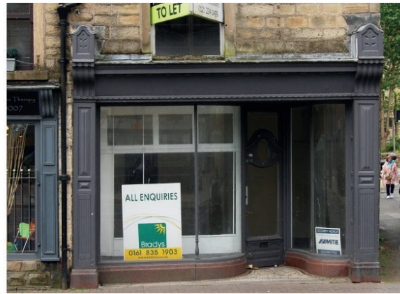
Figure 41: 3 St James Street before
