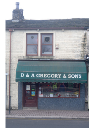
Figure 35: 21 St James Street before
