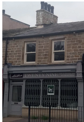
Figure 30: 29 St James Street after
