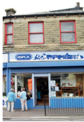
Figure 28: 33 St James Street before
