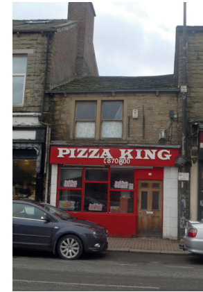
Figure 36: 15 St James Street before
