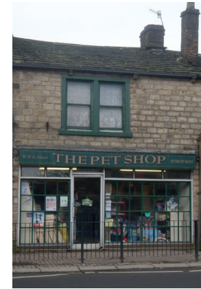
Figure 32: 25 St James Street before
