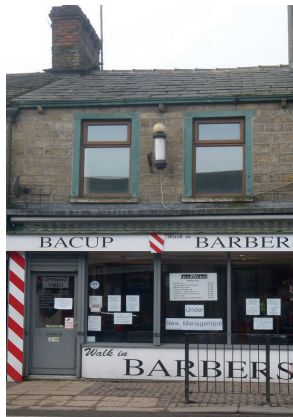
Figure 30: 29 St James Street before
