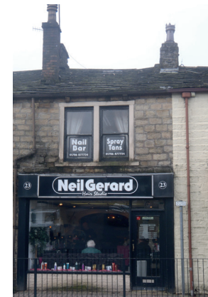
Figure 33: 23 St James Street before
