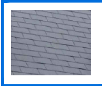
ROOFS TO HOUSES artificial slate - agreed sample
