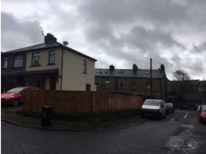
Photograph 1: Elevated position of property and location of proposed extension
