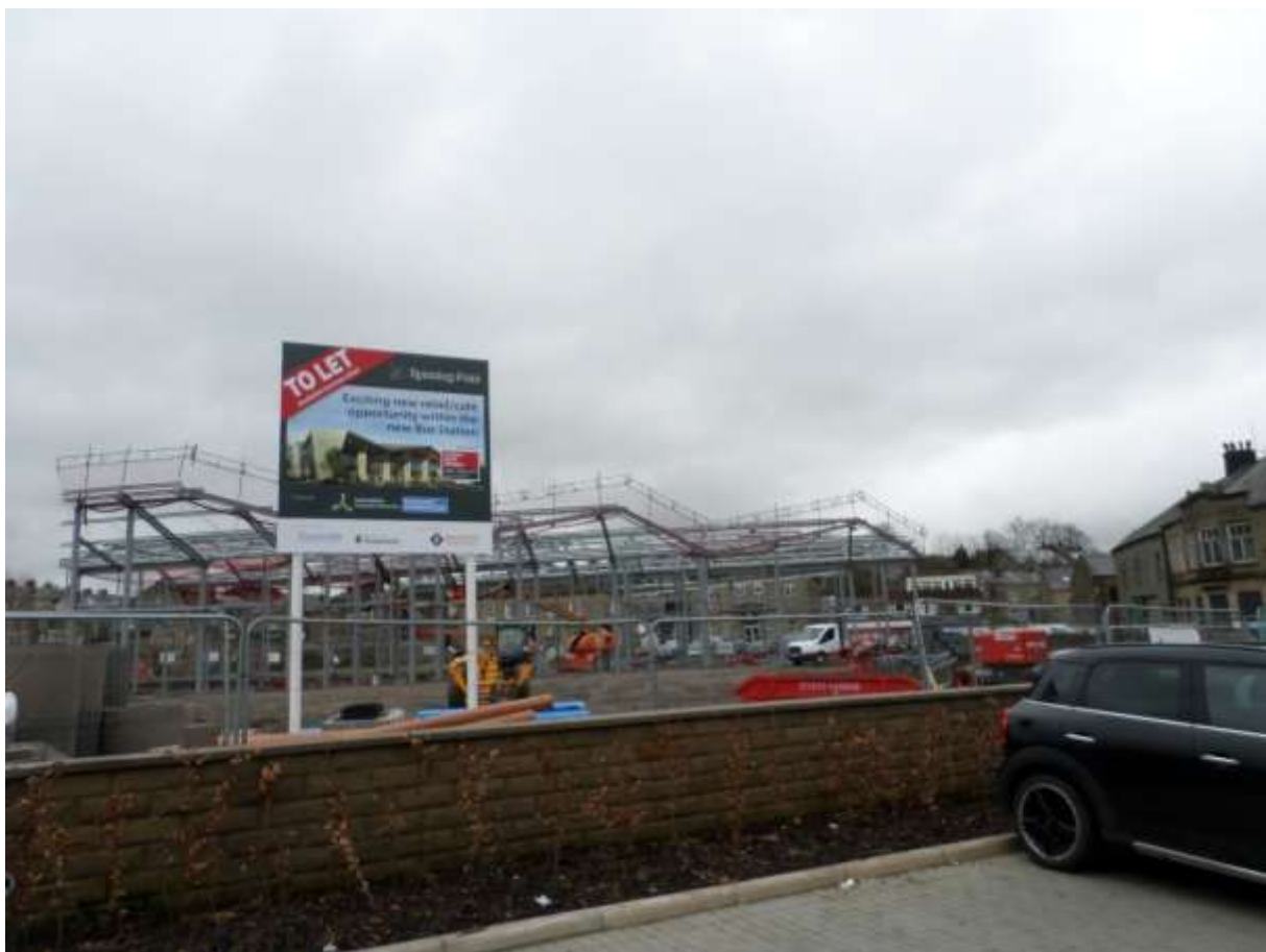
Photograph of the new bus station under construction in March 2019
