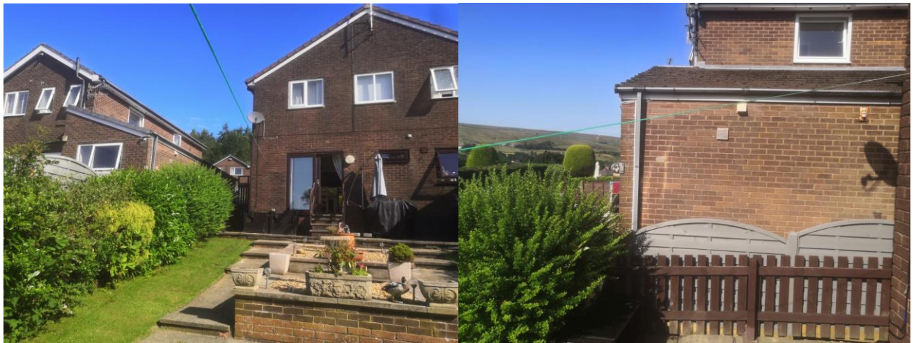
Rear Garden views looking towards No.11
