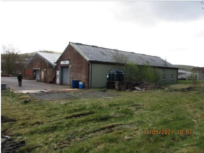
North west facing corner of buildings.
