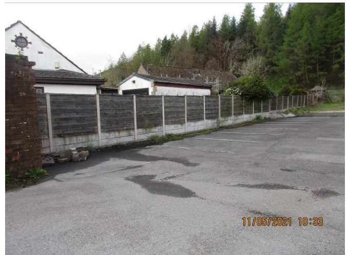
Car park to south end.
