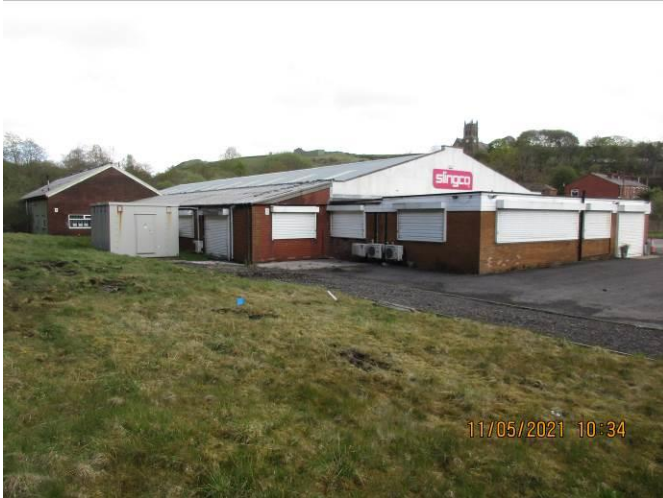
Front elevation from the west.
