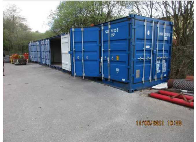
Container yard area.
