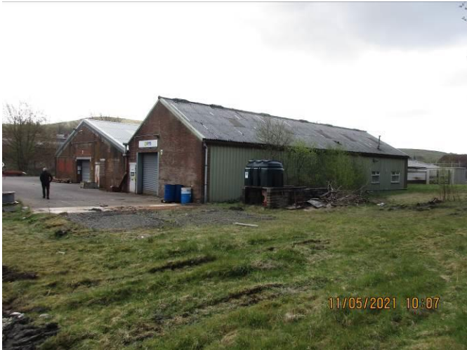
North west facing corner of buildings.
