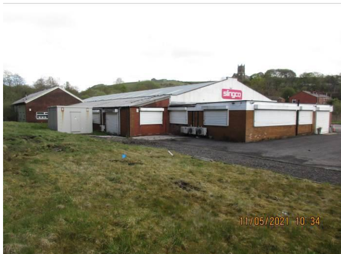
Front elevation from the west.
