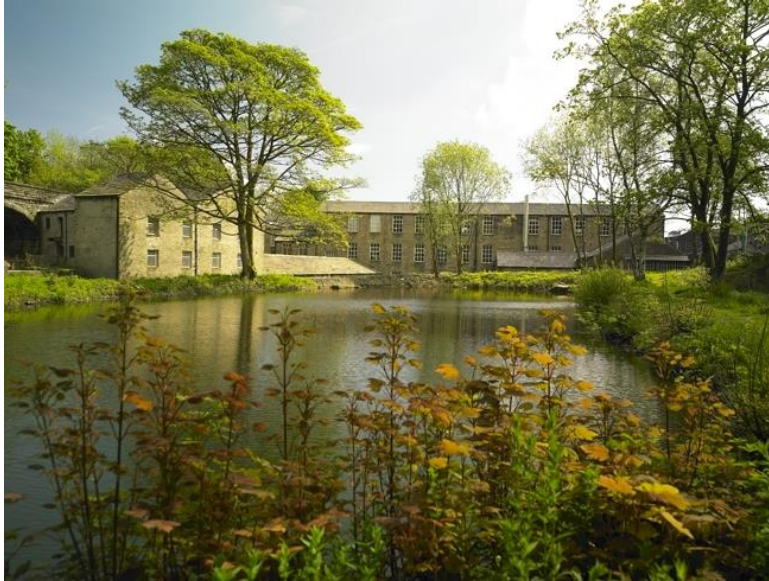
Figure 4 -Helmshore Textile Mill. Source: Rossendale Borough Council Corporate Photo Bank
