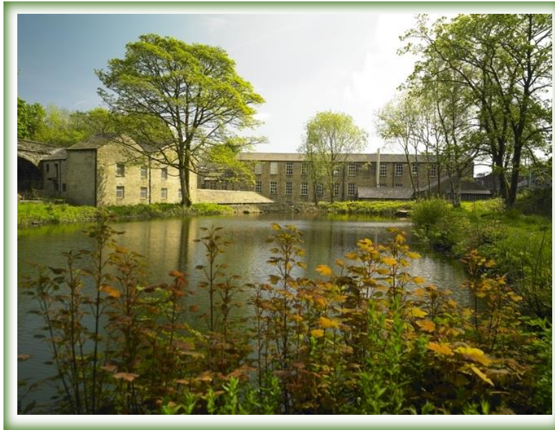
Figure 4 - Helmsshore Textile Mill. Source: Rossendale Borough Council Corporate Photo Bank
