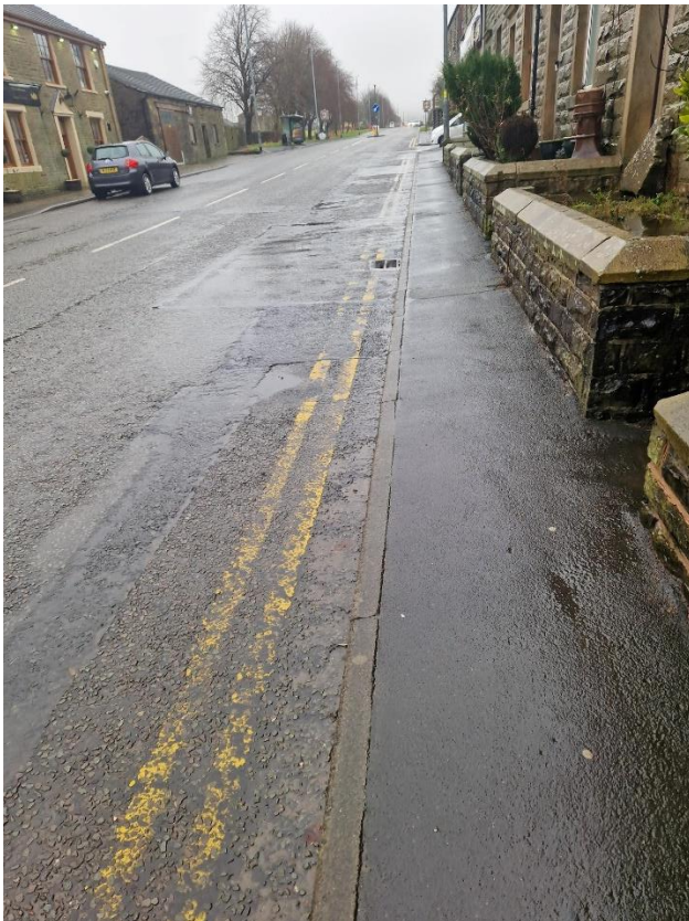
View Northwards to application site
