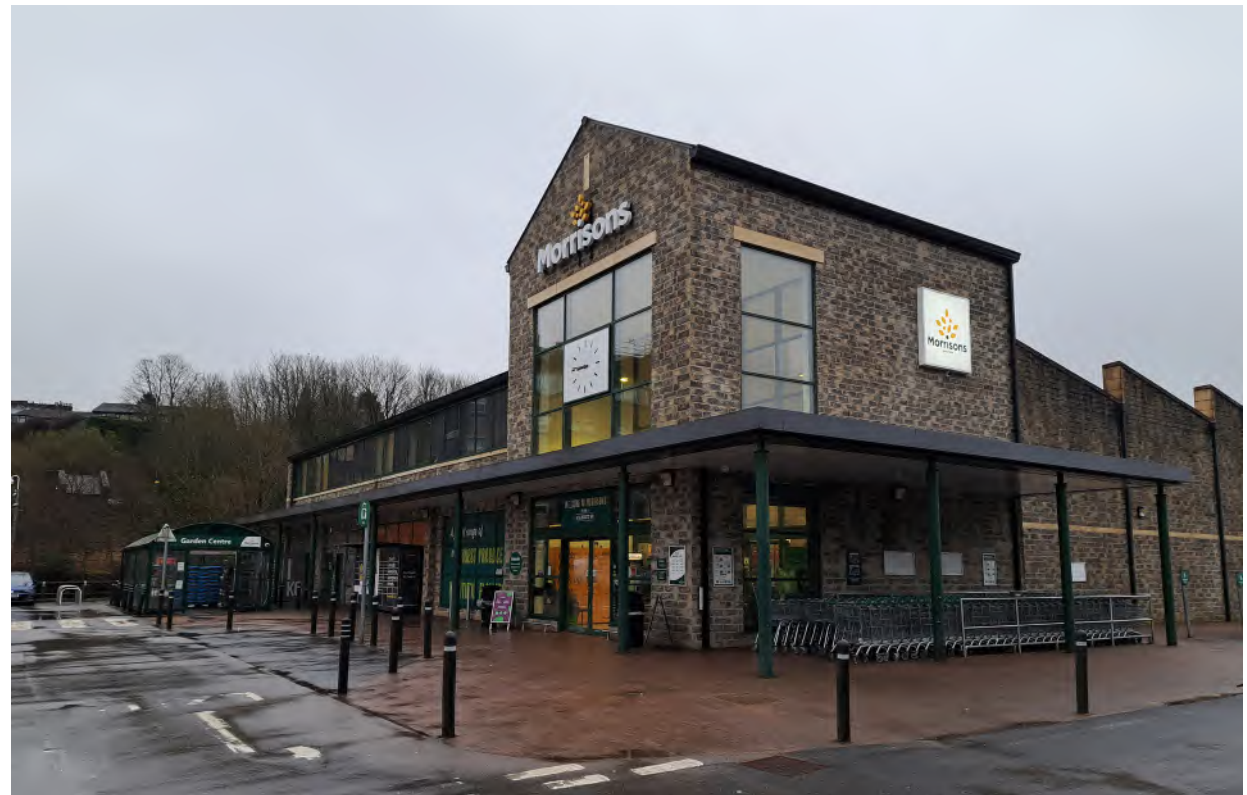
ADJACENT MORRISONS SUPERMARKET
