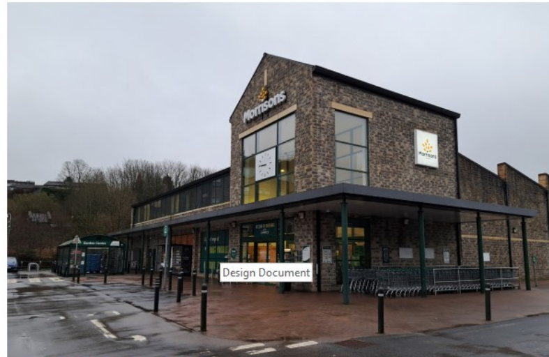
ADJACENT MORRISONS SUPERMARKET
