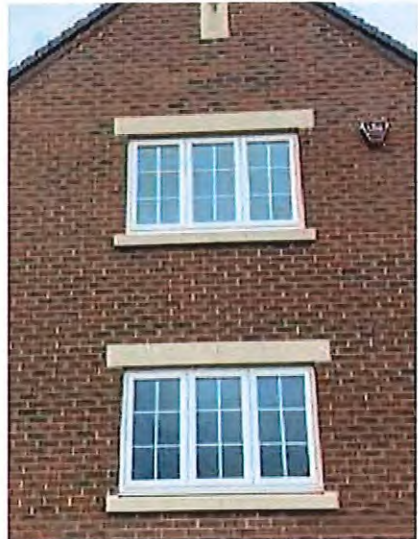
Stone cill and header detail
