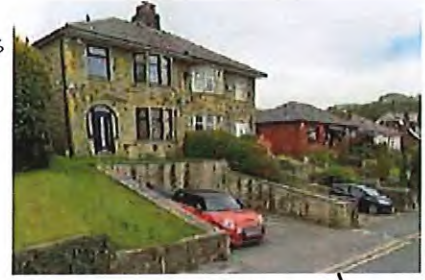
Stone faced retaining walls
