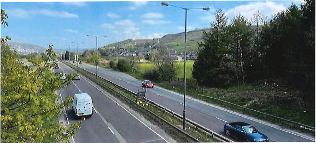
A56 - dual carriageway
