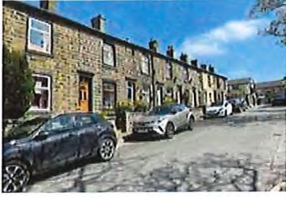
Strong build line along Exchange Street
