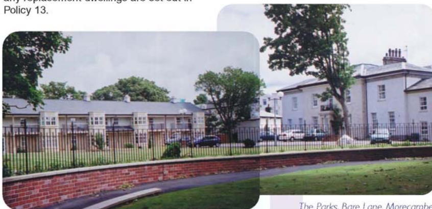
The Parks, Bare Lane, Morecambe commended for Best Urban Regeneration Project by the Royal Town Planning Institute in 2001.
