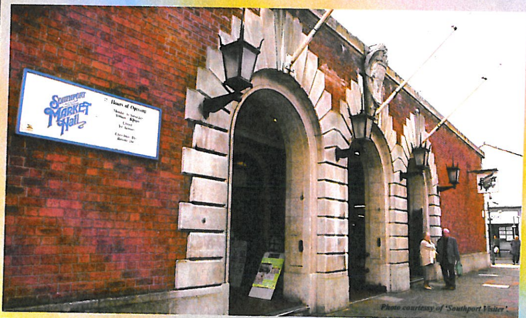
The refurbishment will include modernisation of both the exterior and interior of the Market.
