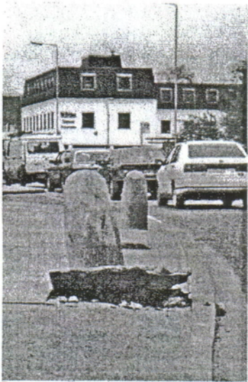
Damage to Bollards
