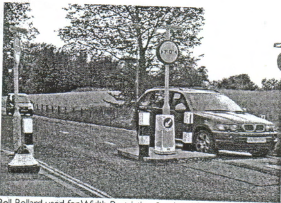
Bell Bollard used for Width Restriction & painted for increased visibility
