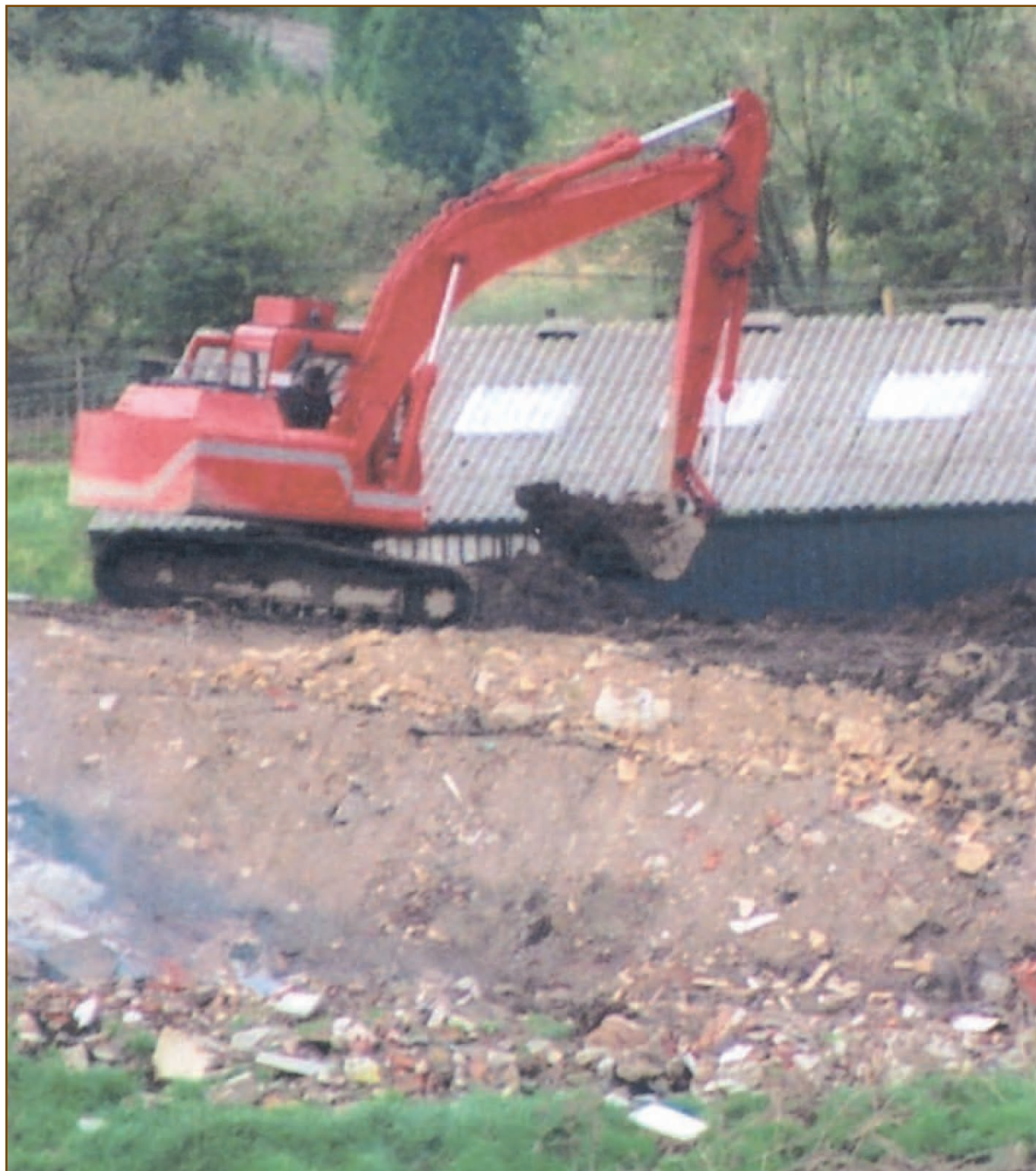
Photograph of excavation on neighbouring land (paragraph 51).
