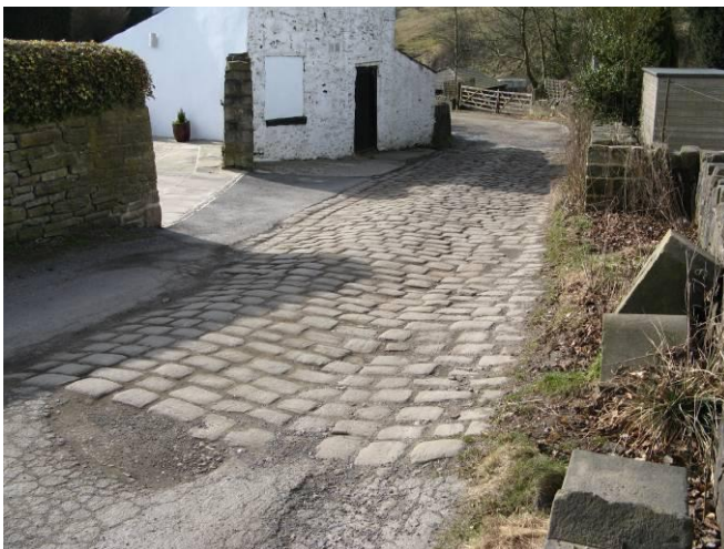
Traditional paving in Goodshawfold
