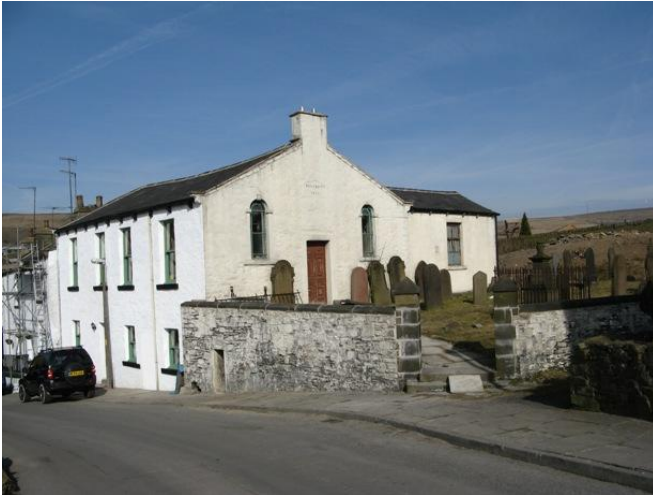
The former Rehoboth Church
