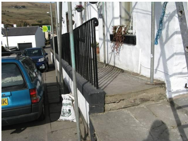
Raised pavement in front of Nos. 13-25 Goodshawfold Road
