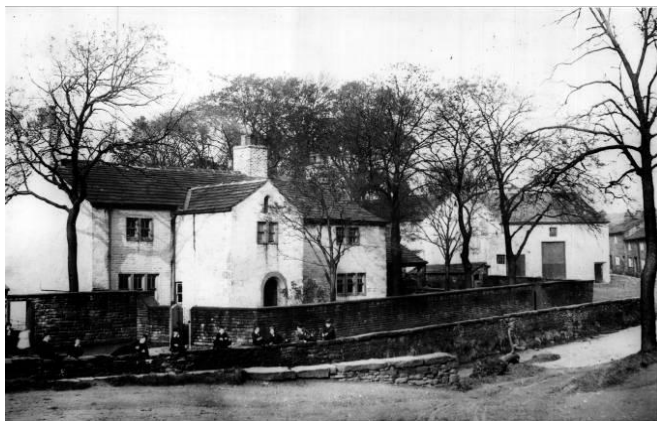
Historic Photograph of Farmhouse and Barn
