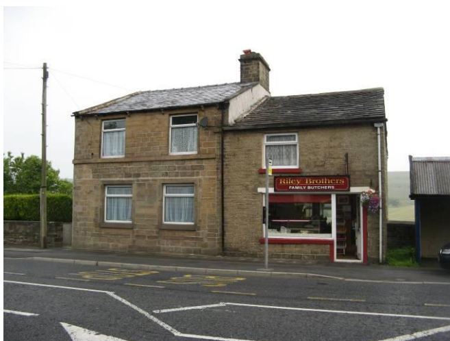
Nos. 1218 and 1220 Burnley Road
