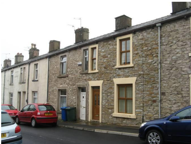
Properties in Commercial Street
