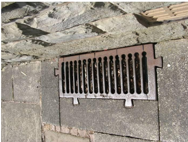
Cast iron grille in pavement in Church Street
