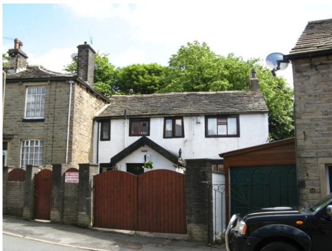
Stone slate roofs in Church Street
