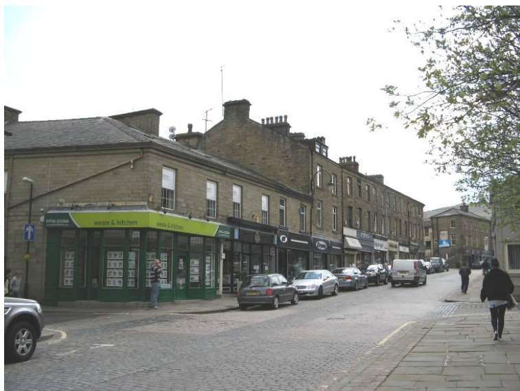
Bank Street looking south
