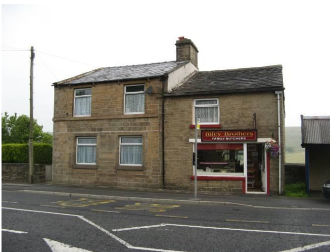
Nos. 1218 and 1220 Burnley Road
