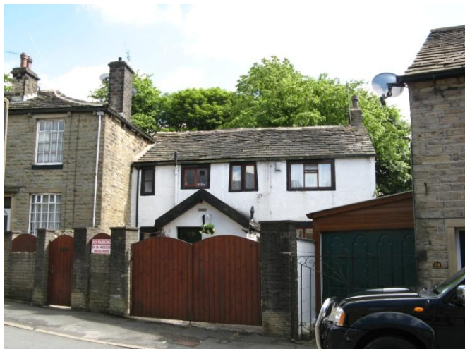
Stone slate roofs in Church Street
