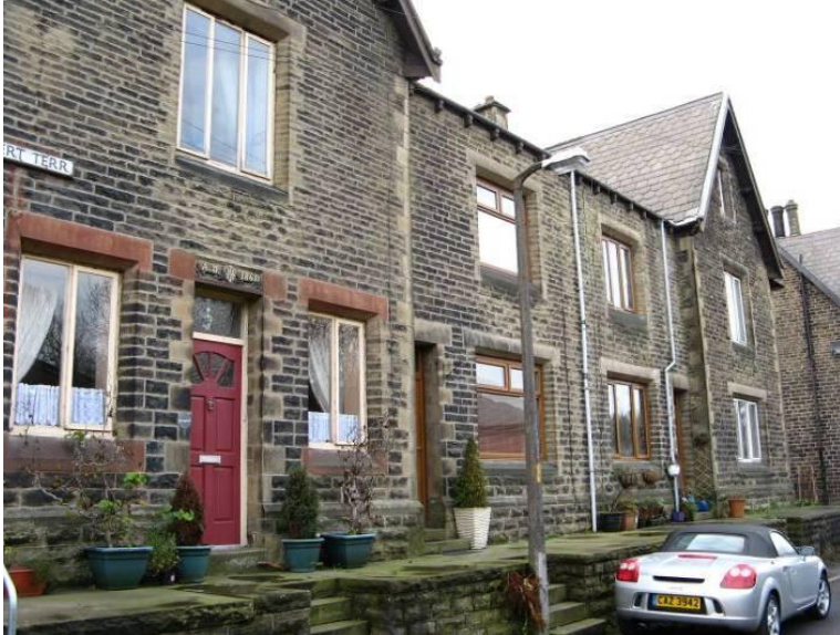
Detail of Albert Terrace
