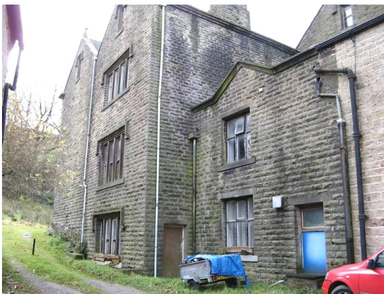
Nos. 3 and 5 Dam Top
