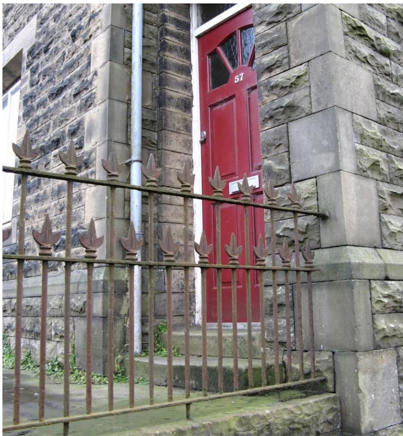
Railings in front of Albert Terrace
