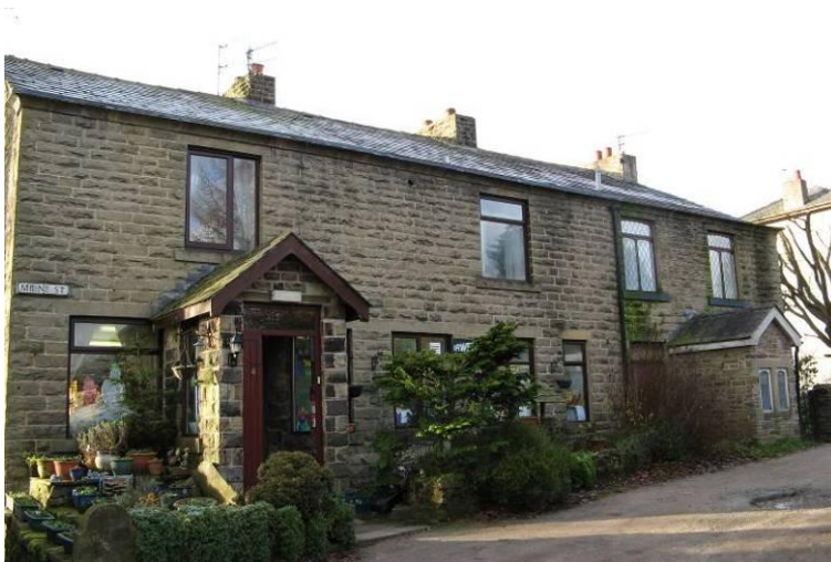
Protect these unlisted properties in Milne Street with a new Article 4 Direction
