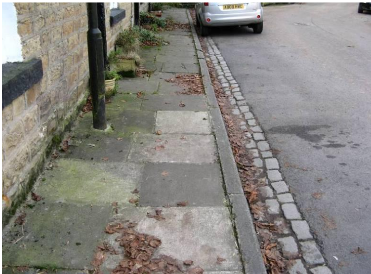
Bowker Street paving
