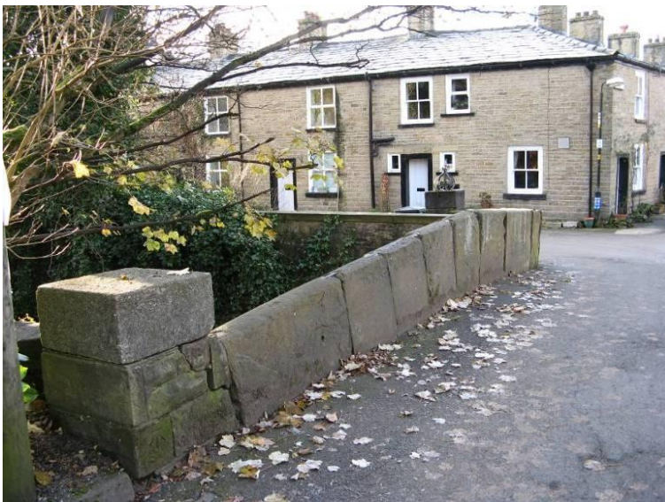
Flag-stone detail on Ogden Bridge
