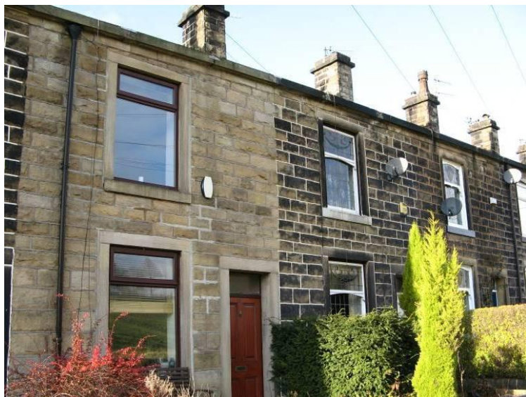
Satellite dishes in Chatterton Road
