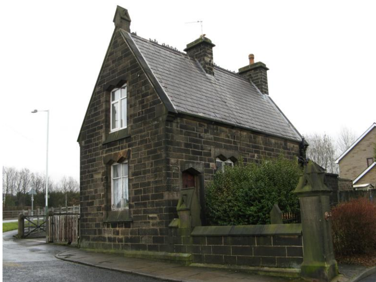
The old School-keeper's house
