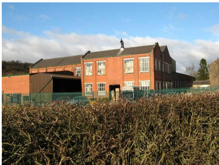
Former mill buildings off Chatterton Road, now used as a furniture warehouse
