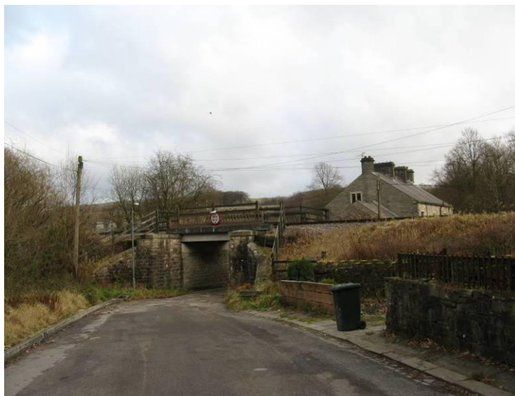
Former railway bridge, Strongstry
