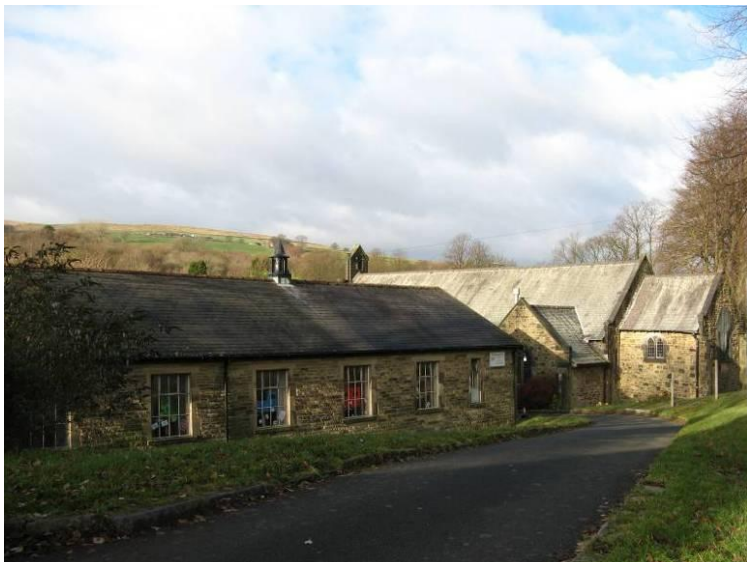
St Philip's Church and the former Sunday School, Chatterton Road
