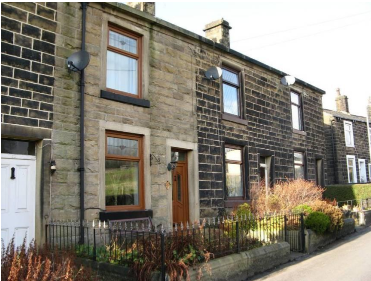
This house (No.93) in Chatterton Road has been cleaned
