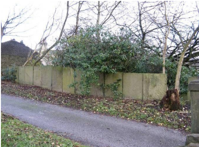
Sandstone paving slabs used as boundary next to No.422 Newchurch Road
