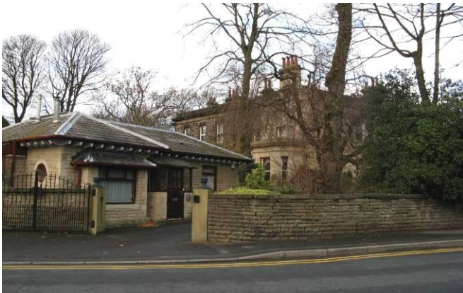
Springhill House and its lodge facing Newchurch Road
