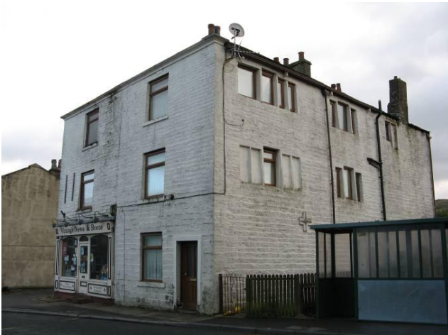
Nos. 423, 425, 427 and 429 Newchurch Road
