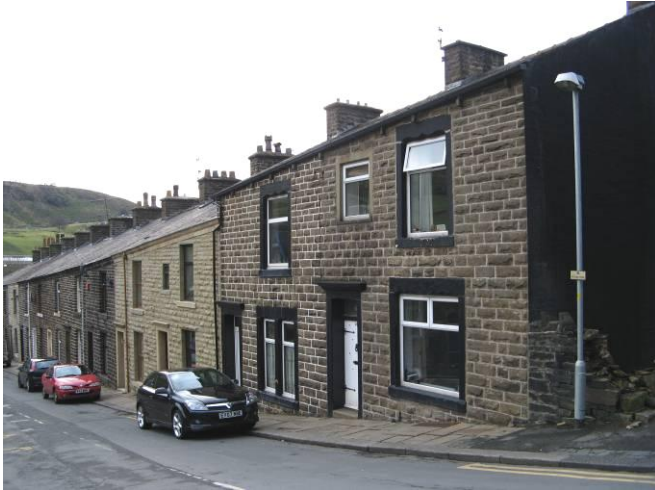
Part of Peel Street Terrace (Nos. 2 – 28 (even))
