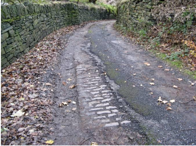
Section of Dobbin Lane paving
