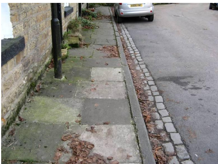
Bowker Street paving
