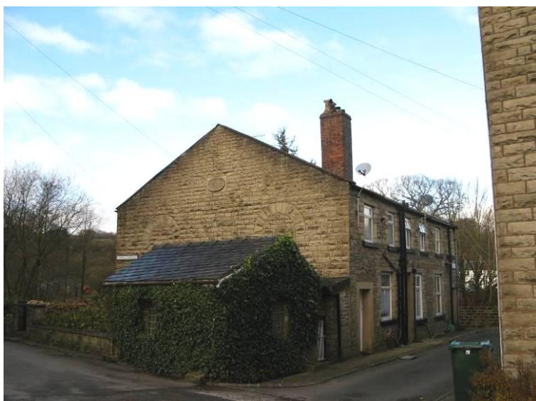
The former Primitive Methodist Chapel, now three cottages
