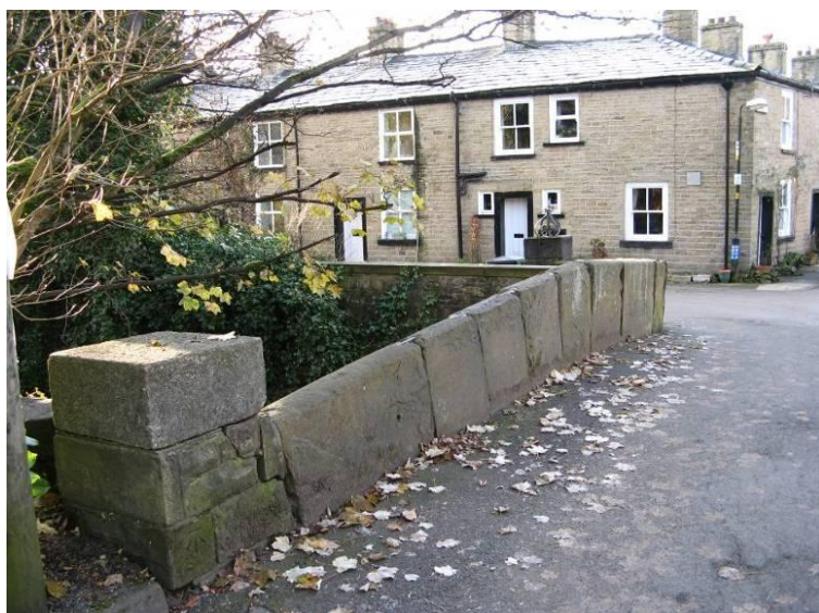
Flag-stone detail on Ogden Bridge
