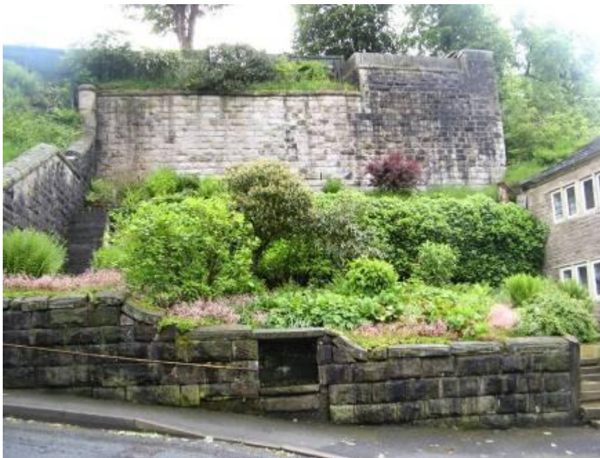
Boundary wall in Bankside Lane
