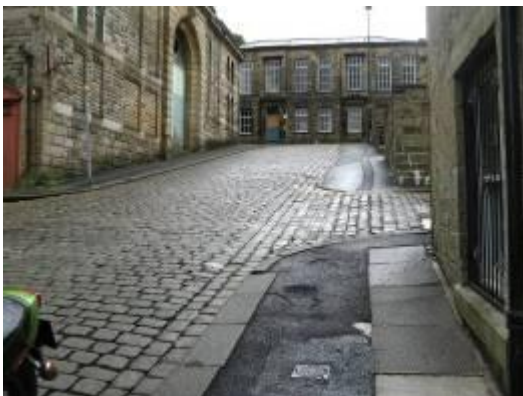
Traditional paving in Bank Street although the stone pavements have been replaced
