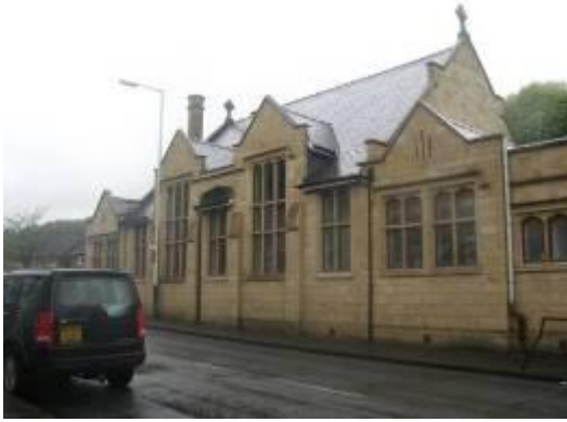
Former Sunday school, Burnley Road
