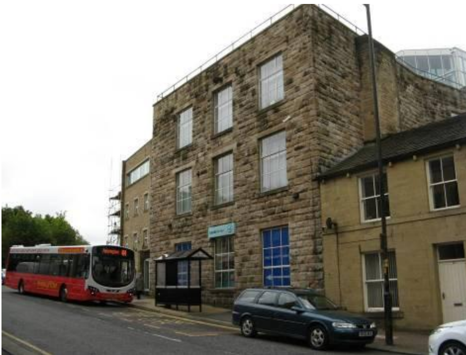
Irwell Mill, from Rochdale Road
