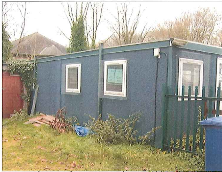
TYPICAL PORTAKABIN ACCOMMODATION
