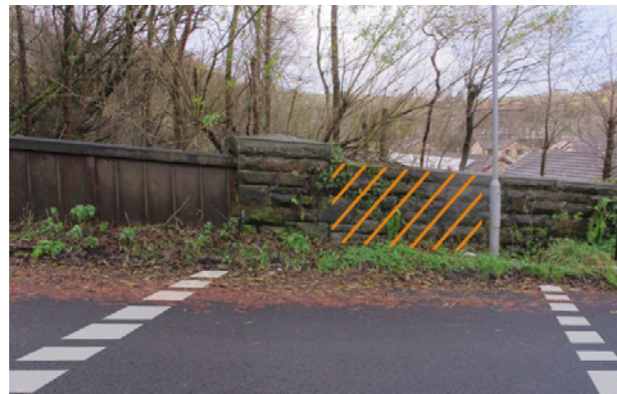
Rakehead Lane showing the proposed entrance to be made through the railway boundary wall just downhill of the remaining bridge parapet. These bridge parapets will be attractive features clearly visible from the path approach on either side. They could be painted in the project colours
