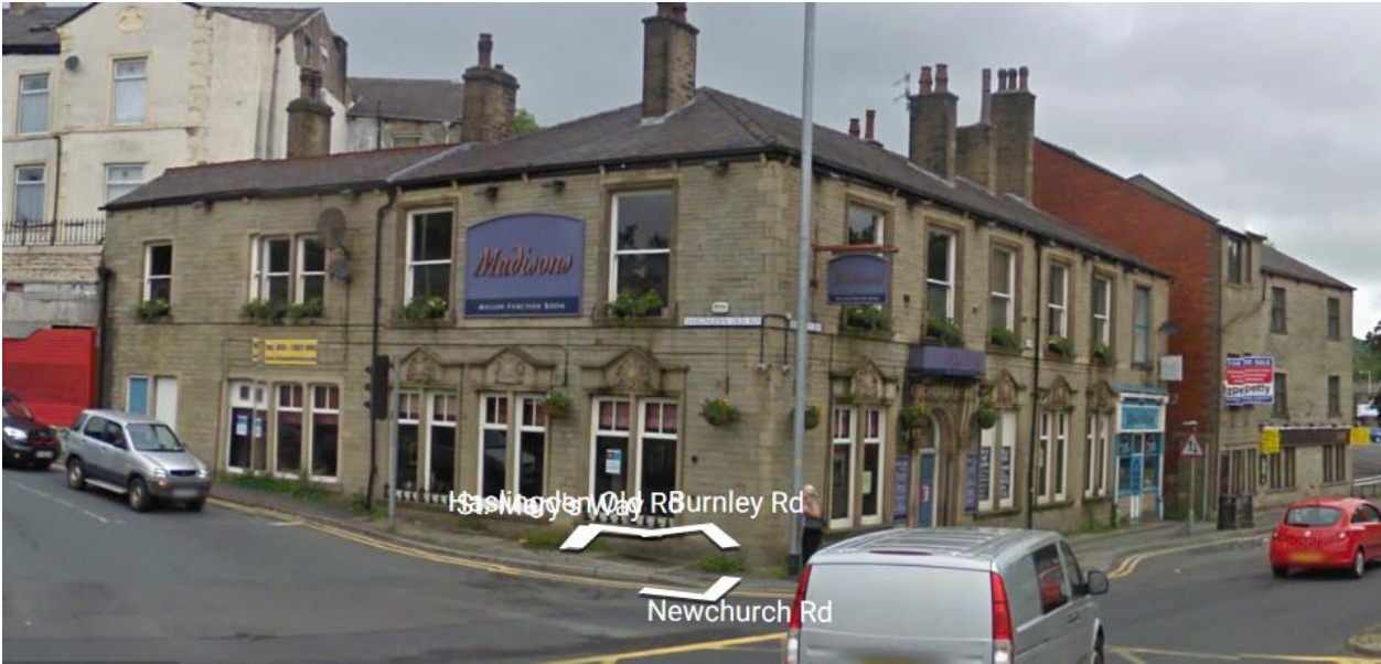
Building prior to renovation
