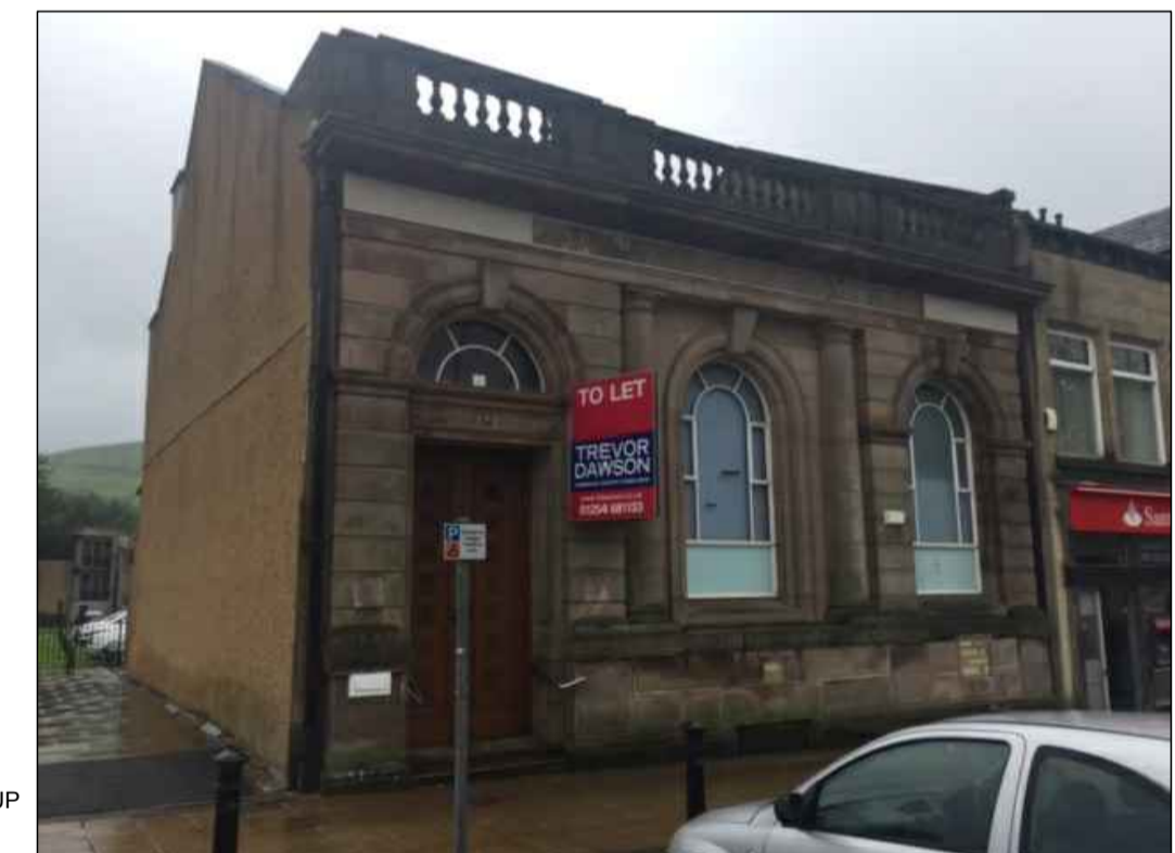
EXISTING PHOTO B
