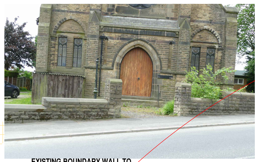
EXISTING BOUNDARY WALL TO ROCHDALE ROAD RETAINED
