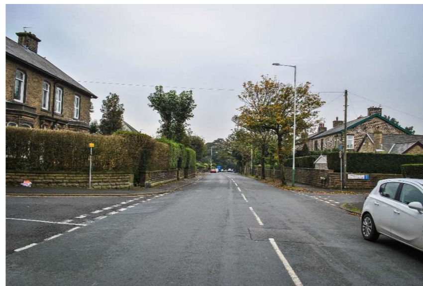
Figure 31 Helmshore Road looking south
