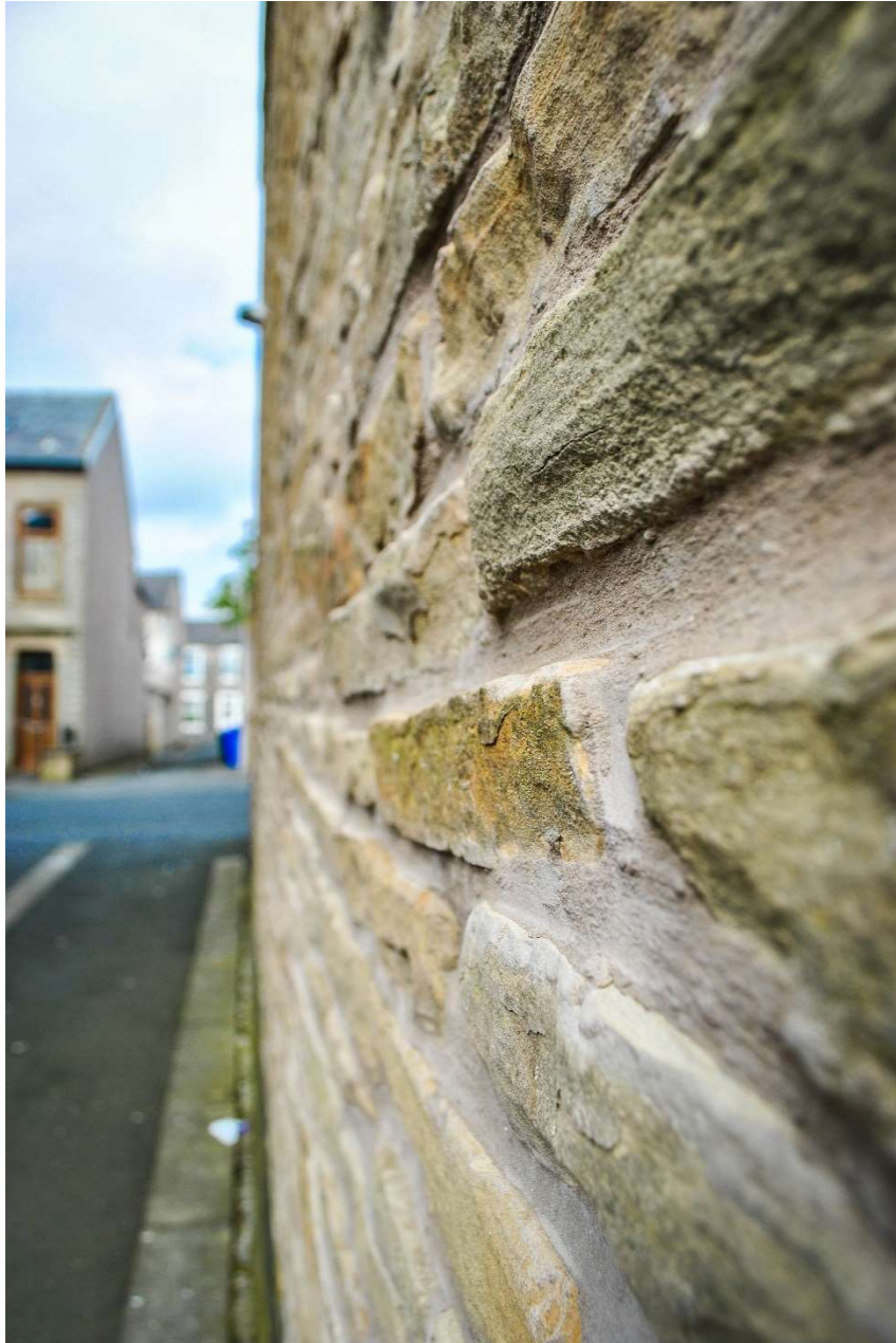
Figure 43 Example of watershot coursing
