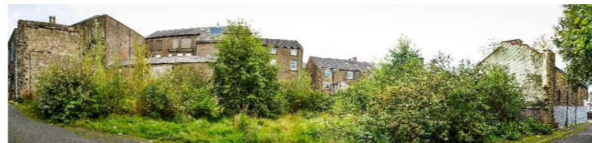
Figure 14 Overgrown, disused space on Bell Street.
