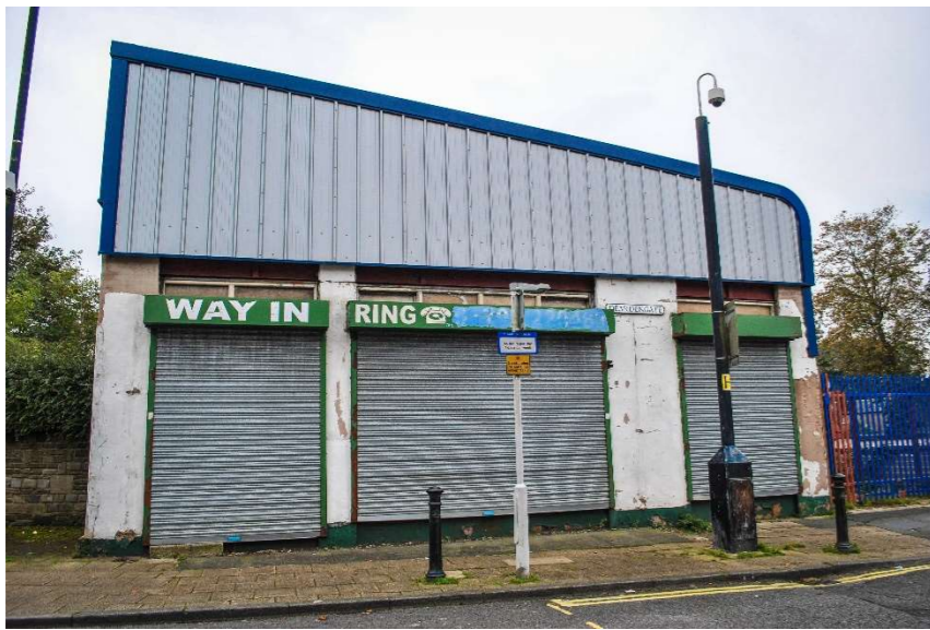
Figure 84 (Disused?) Garage on the corner of Helmshore Road and Warner Street.
