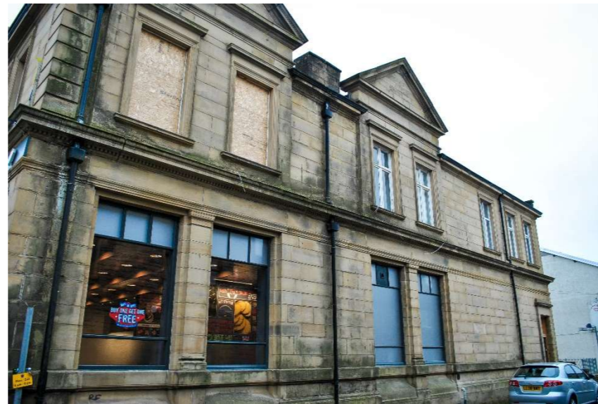
Figure 86 67 Deardengate from Ratcliffe Street
