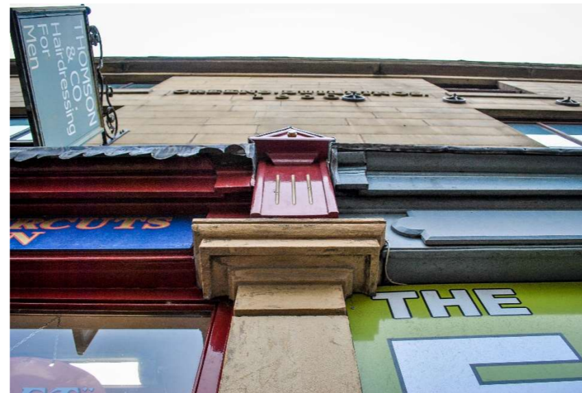
Figure 97 Thomson Barber Shop, 63 Deardengate - detail
