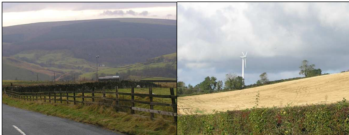
The turbine in the centre of the photo on the left, seen mainly against a dark forested hillside, is very effectively camouflaged by its dark colour; while the pale grey turbine on the right, seen mainly against the sky, blends well with this background in most light conditions.
