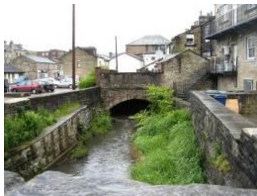
The River Irwell outside Industrial Place
