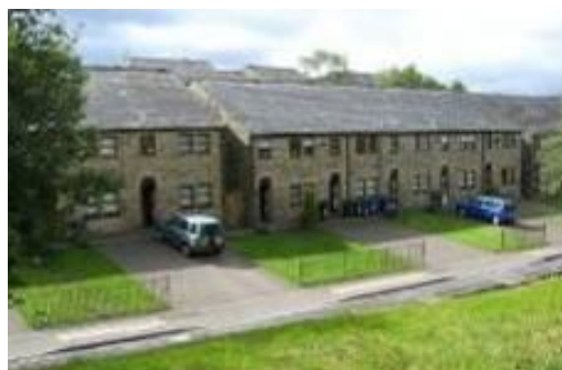
Well designed new housing facing Todmorden Road (on the site of the former Tong Mill)
