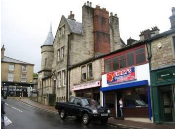
Poor quality shopfronts in Union Street
