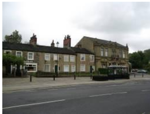
St James Street eastside
