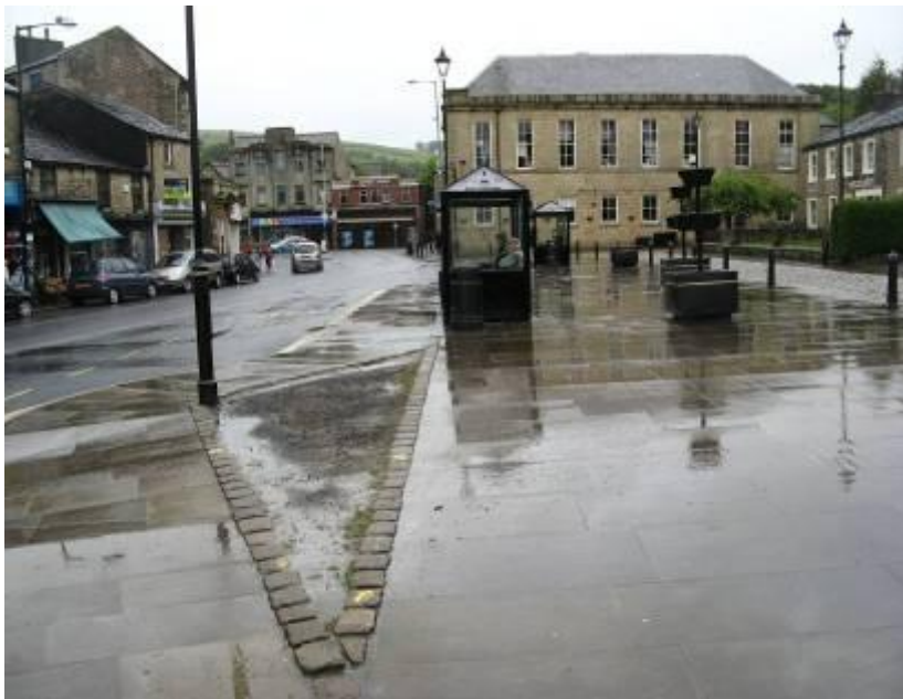
East side of St James Street, showing repaved area
