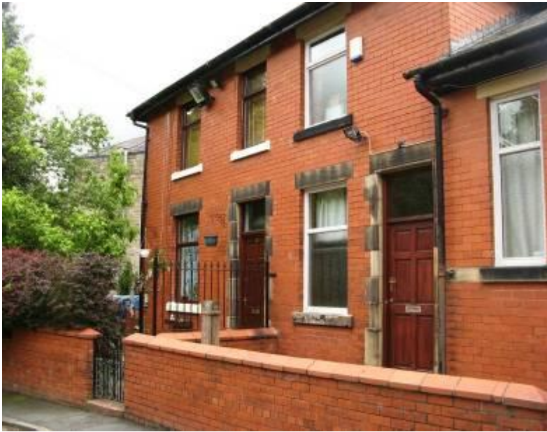
Brick building in Princess Street (No.11)
