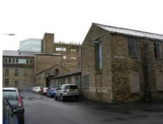
Lee Street, with Irwell Mill at its eastern end, still retains an industrial character
