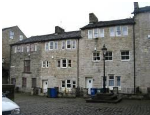
Sash windows in the restored listed buildings backing onto Industrial Place
