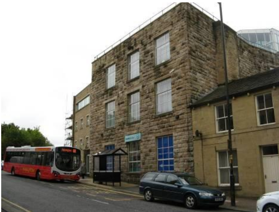
Irwell Mill, from Rochdale Road
