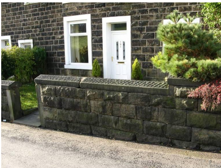
Boundary wall outside No.101 Chatterton Road
