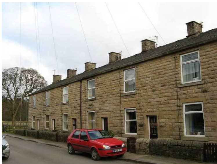
These unlisted buildings in North Street could be protected by a new Article 4 Direction
