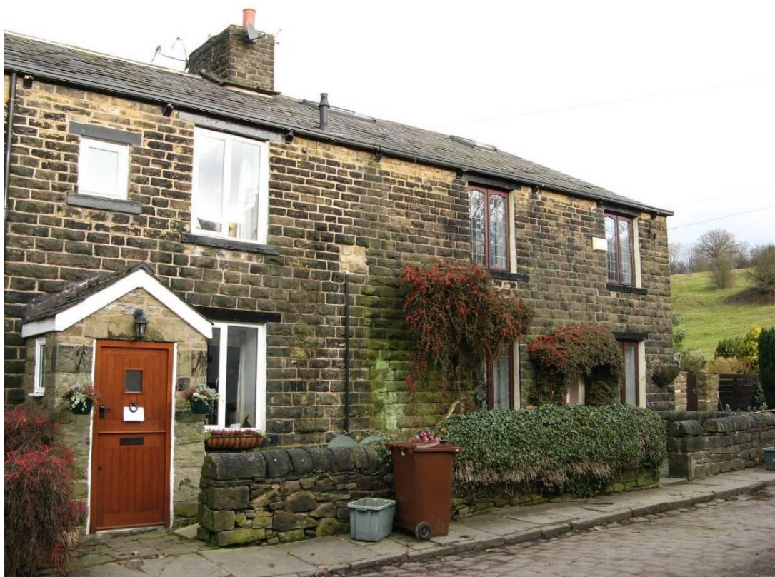
A small porch has been added to this house in The Park
