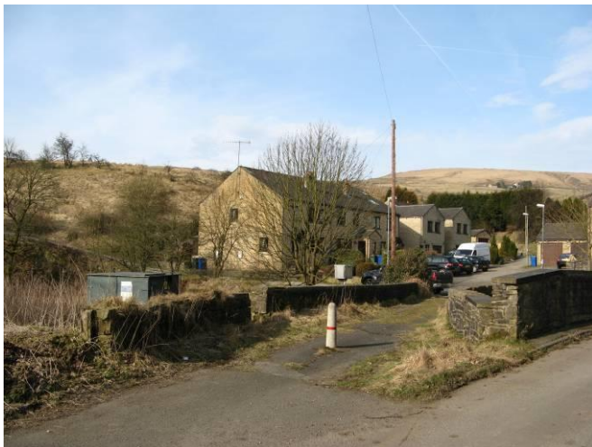
Bridge over the Limy Water
