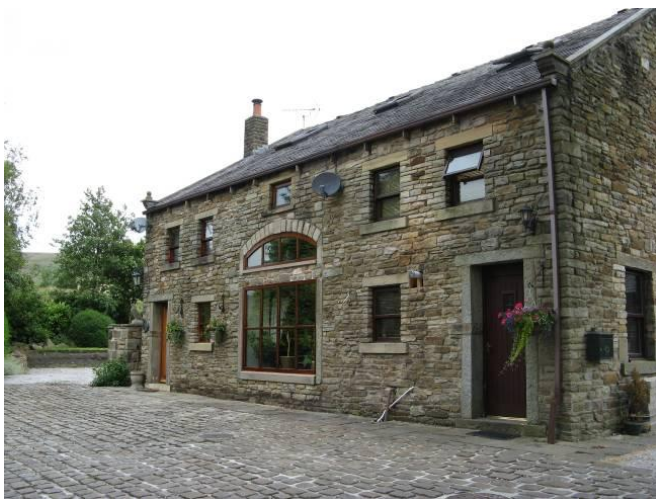
The Old Croft / Cloughfield Barn
