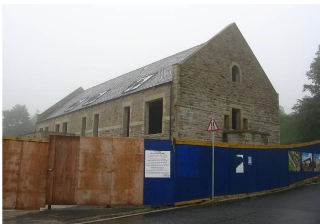
The former Canteen (work has re-started since this photograph was taken)
