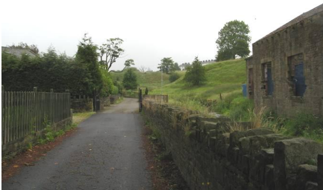
A mixture of boundary details next to the Limy Water
