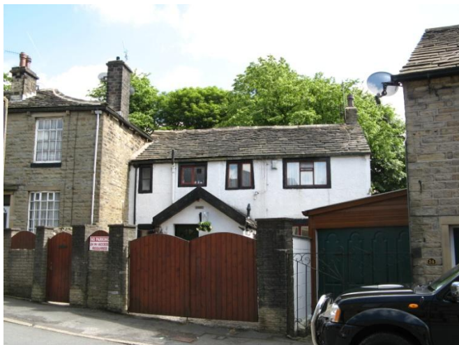
Stone slate roofs in Church Street
