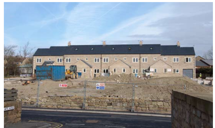
View of construction of Clovercroft
