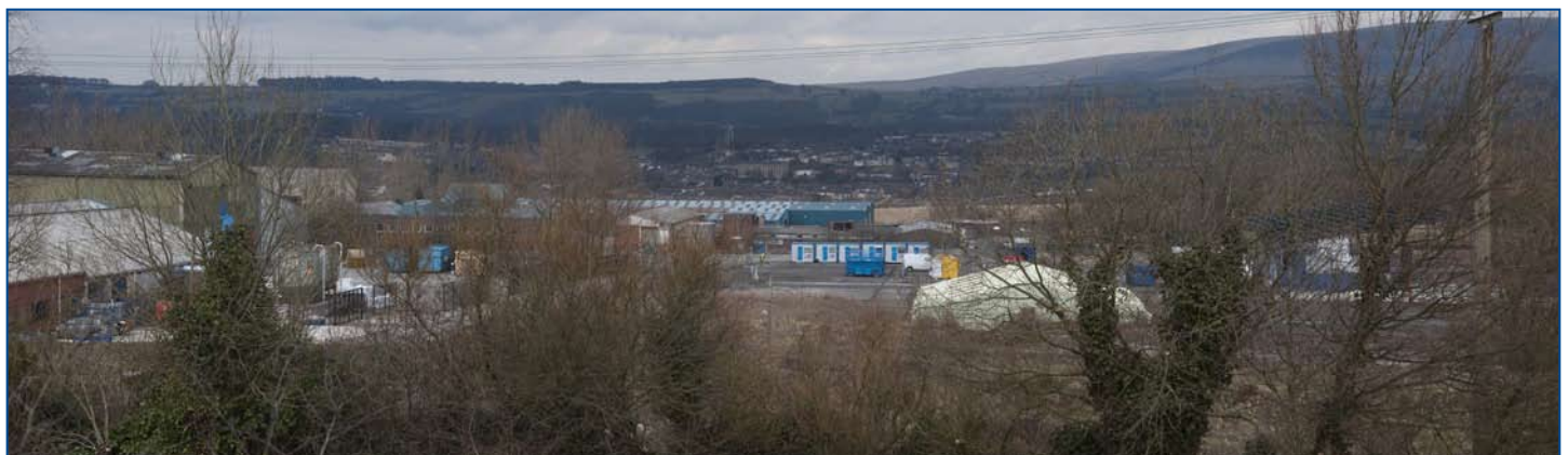
Existing partly demolished site
