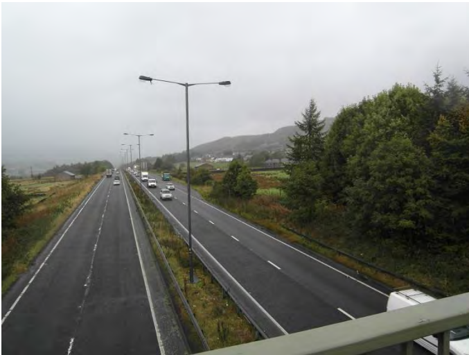
P2 View North from A56 footbridge
