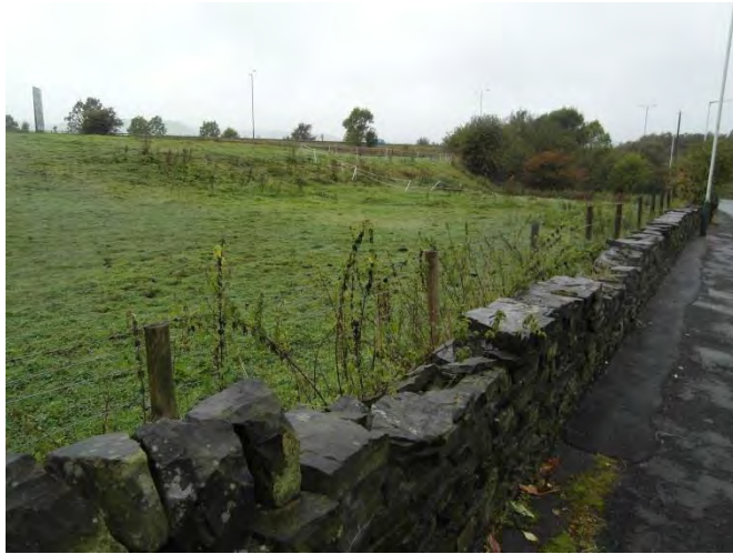
P3 View north west from Blackburn Road
