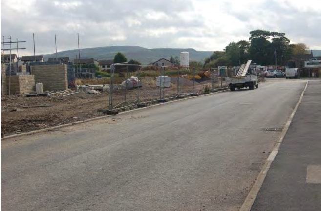
P4 View into building site, looking south along Hollin Way
