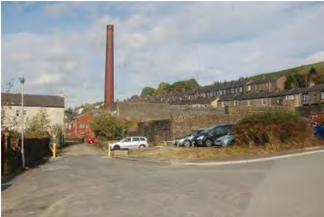
P5 View north from Vale Street looking towards existing industrial buildings
