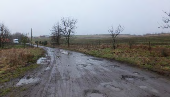
P5 View north along footpath 448 towards Bent House, to left, and quarry right and centre
