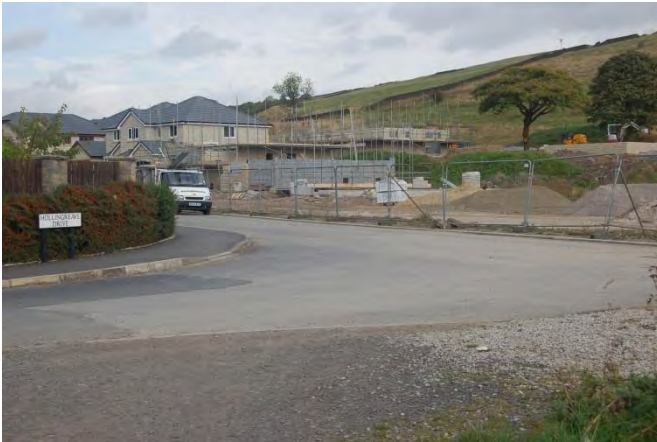
P3 View north east into building site from Hollingreave Drive
