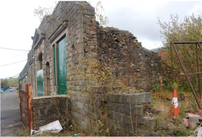
P3 View of façade to mill on Ormerod Street
