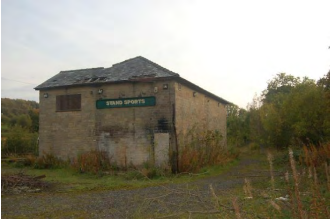
P4 View of derelict clubhouse from the north
