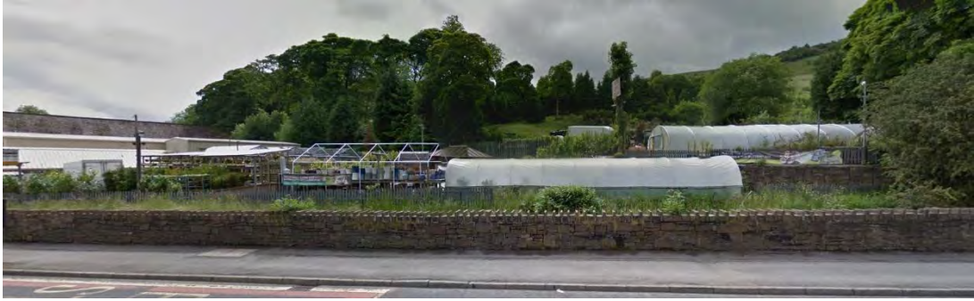
Figure 1.2 The site, viewed from Burnley Road
