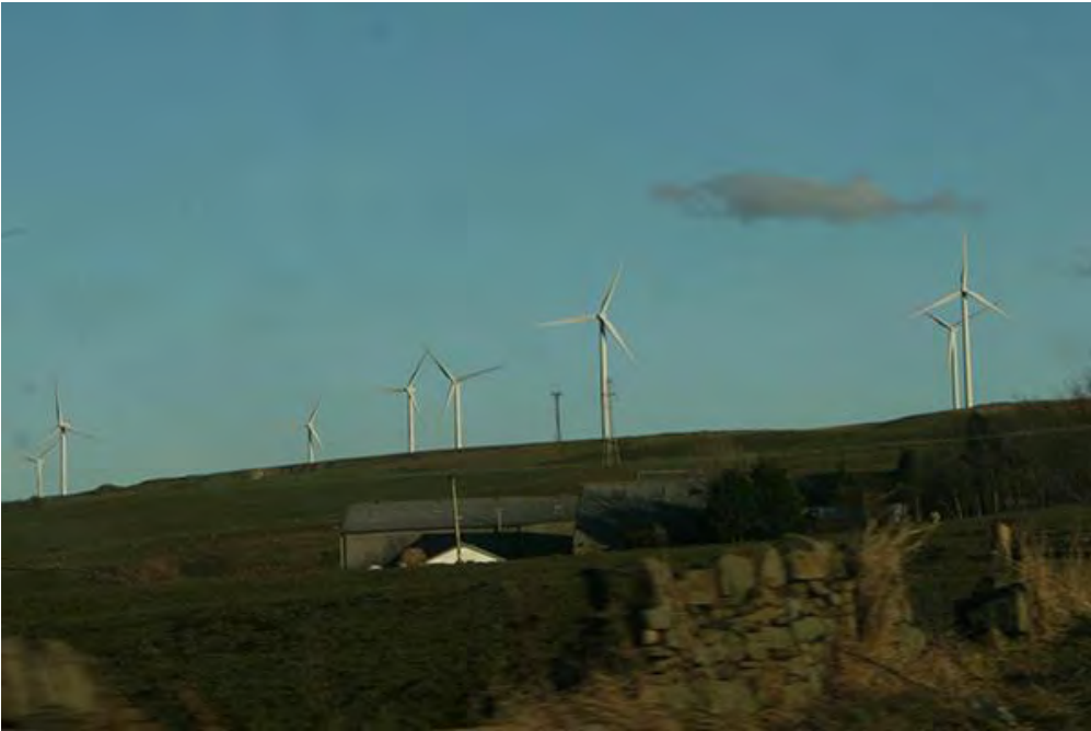
More turbines from Haslingden Moor Wind Farm
