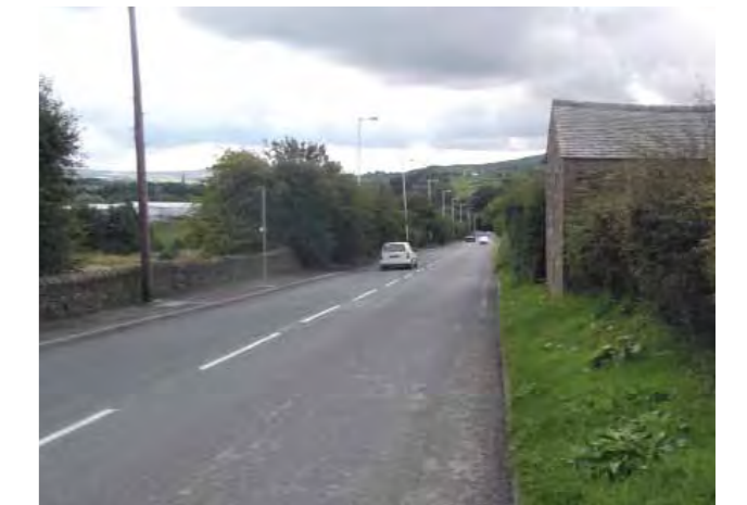
Photo 7: Looking south down Holcombe Road
