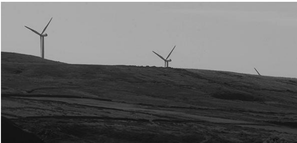
Existing Scout Moor Wind Farm turbine sticking up above the horizon. Photographed from Bacup.
