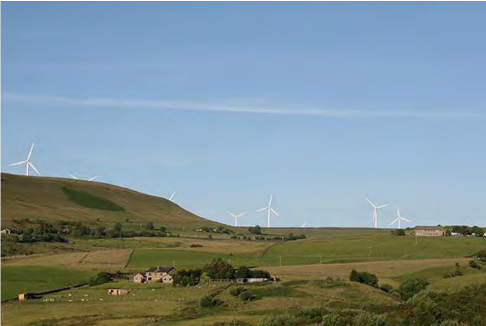
Scout Moor Wind Farm from public footpath.
