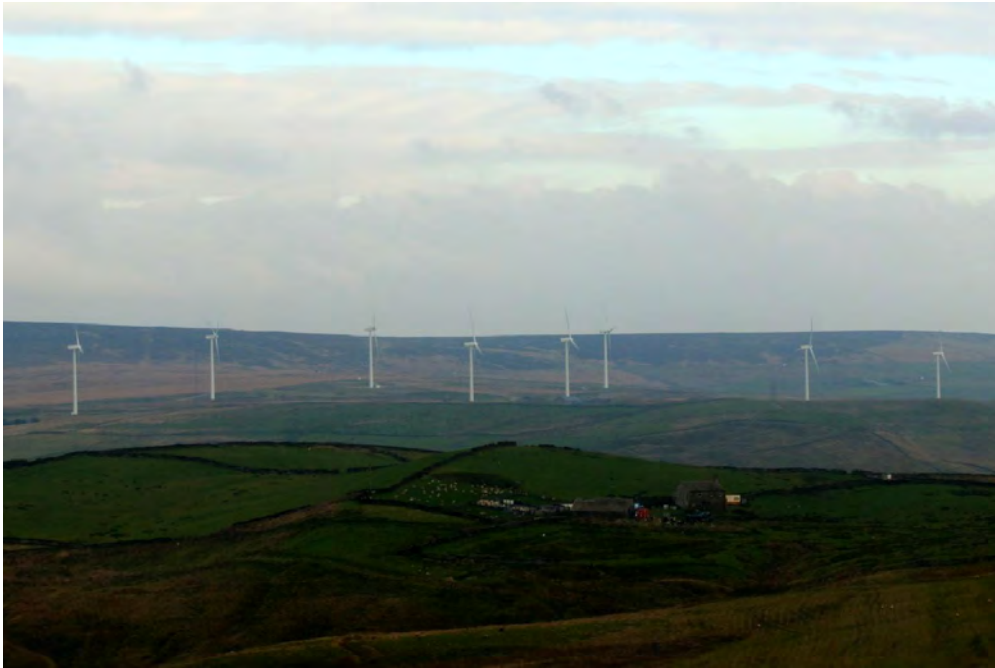
Cliviger Wind Farm photographed from Crown Point.
