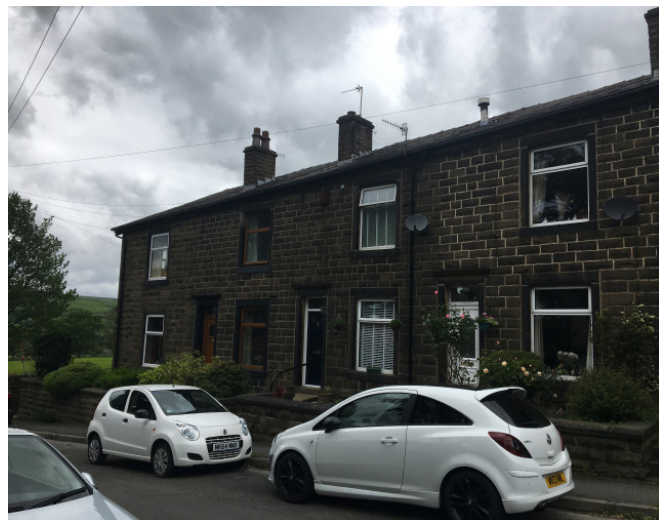
Terraced houses on Exchange Street
