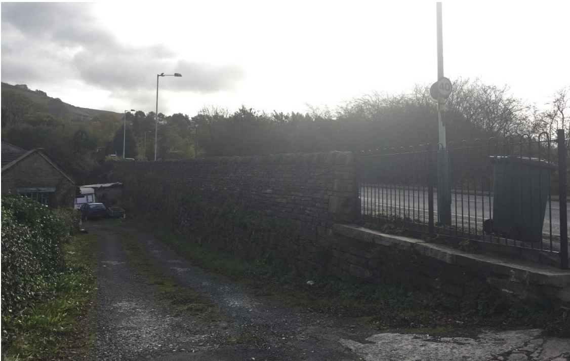
Figure 2: Existing stone wall east of proposed access road
