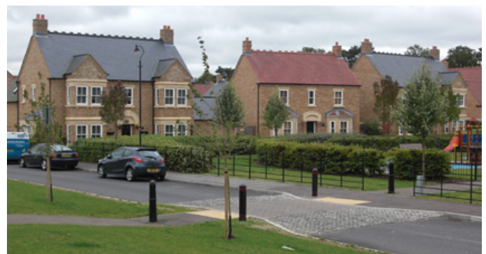
At Fairfield Park in Bedfordshire, vertical calming and 'pinch points' remind drivers they are in a 20mph zone
