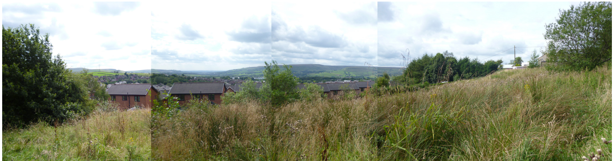
View south west across valley and existing housing from upper slopes of site A
