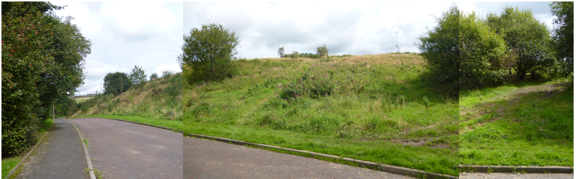
View north along Moorland Rise towards steep embankment on eastern side
